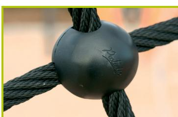
12-**The cables** are linked together and held in place by injected polyamide spheres.
