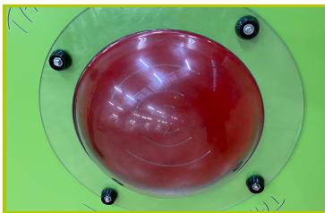
8- **The dome** is made of 3mm polycarbonate sheets.
