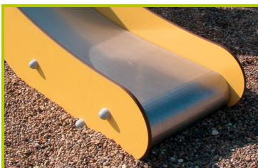
**7- The sliding surfaces** are made of 2mm thick stainless steel, which is shaped, bent and rolled from one piece.
