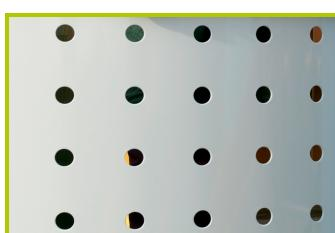
5- **The tunnel**, is made of 3mm perforated aluminium sheet, coated with polyester epoxy lacquer, 427mm in diameter.
