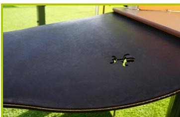
**9- The gangway floor** is made of a woven strip with rubber surface.
